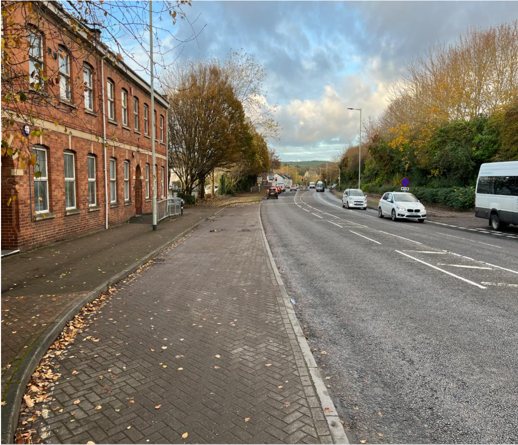
The Site viewed from Alexander Road looking towards its junction with Bear Street.
